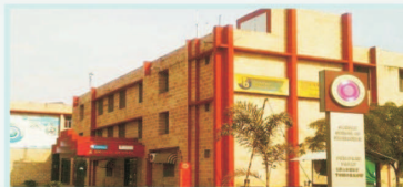
SANGAM SCHOOL OF EXCELLENCE Elementary to Class 12 Residential Day Boarding CBSE & IB World School
